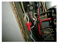
Screws that secure the panel cover to the panel box are missing. This is a potential hazard. Missing screws should be replaced with the original style blunt end screws.
