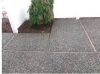
When the wooden dividers separating the concrete walkway sections have deteriorated to a point where they become a trip hazard. Replacement with mortar is recommended.
